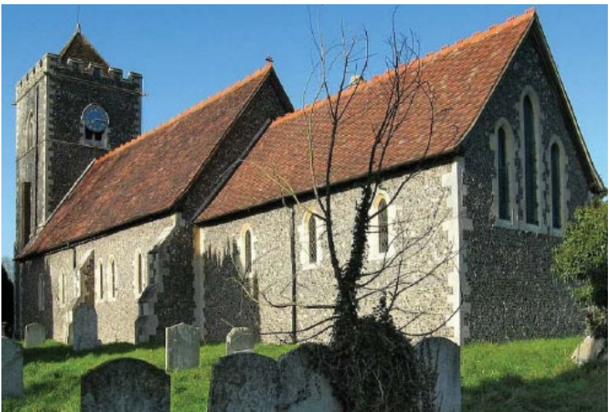
Fig.48 St Botolph's Church flint walls and clay tiles
