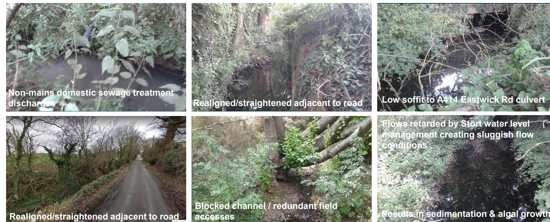
Fig.94 Hydrology engineers analysis of on-site conditions
