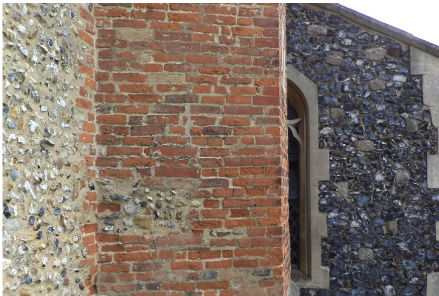
Fig.47 Flint and clay brick on St Mary's Church
