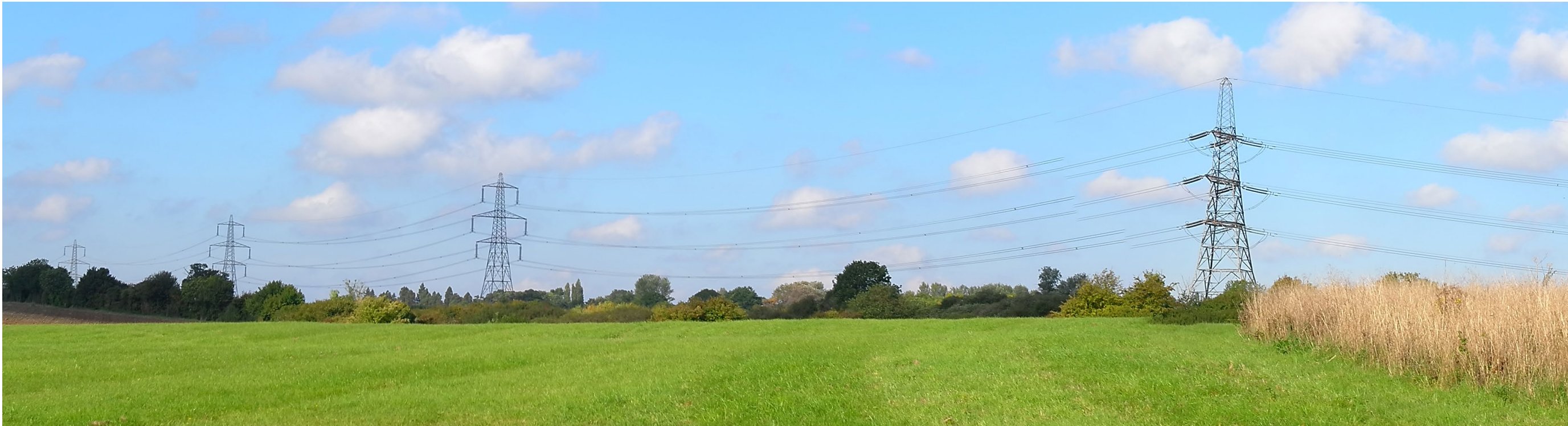
Fig.91 High Voltage transmission lines to the west of Home Wood looking towards the future village 7
